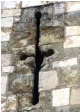
Figure 2 shows the large slit used when firing the Springald from inside the gate tower.
